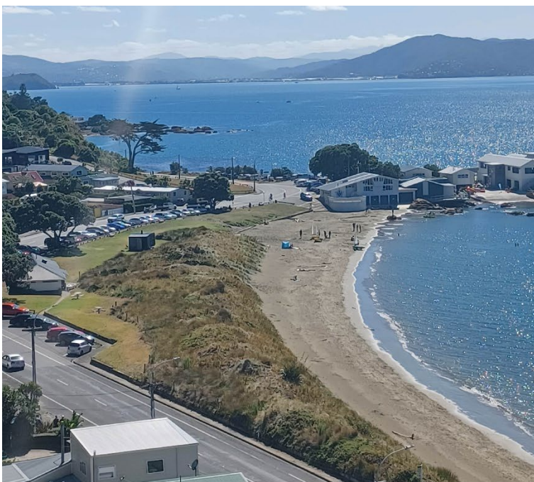
Current situation at Worser Bay showing the extent to which the back (western edge) of the dune is starting to engulf the pavilion and the amount of grass that is now covered by dune
